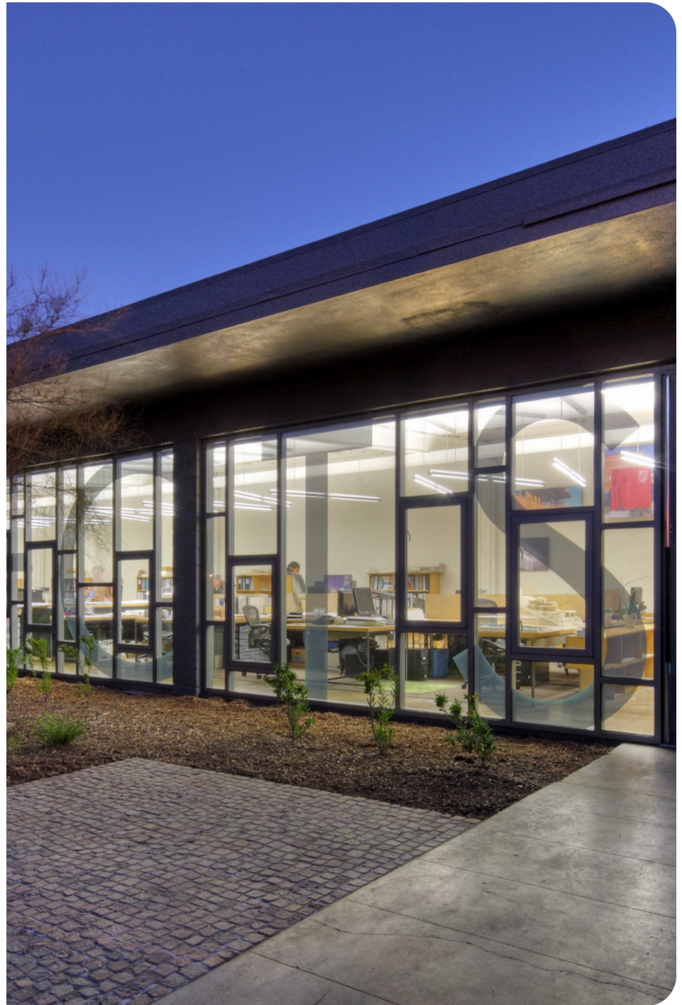
Architects HGW transformed a former gas station and auto repair shop into California's first net-zero-energy building with the help of Solarban® 70 glass by Vitro Architectural Glass (formerly PPG glass).
